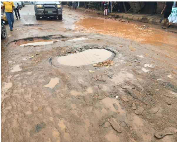
Plate 1: Failed road portion Technical college road plate2: Failed road portion Textile mill road
